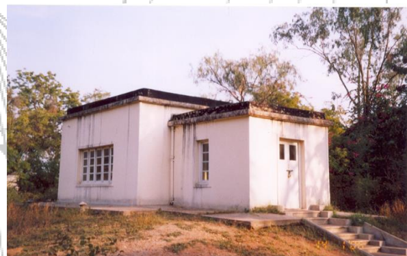
Fig. 2.1c: Secondary variometer building
